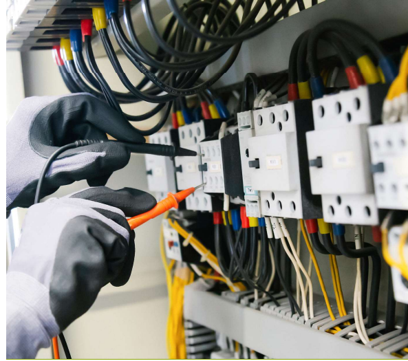
DG Set Power Backup
